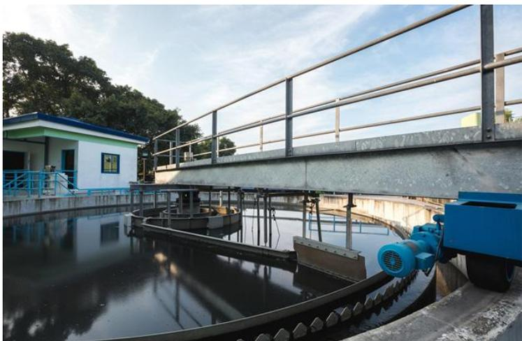
The Tandang Sora STP, which uses an STM-Aerator combining activated sludge and fixed film technology in a compact biological treatment system.
