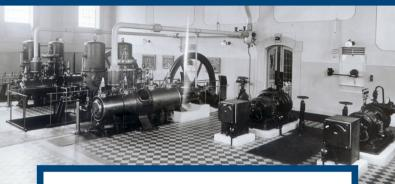
The Kőbánya pump house, established in 1903 to support the water supply of the East-Pest upper zone, utilized the technology of its era and received steam-driven piston pumps. 4 groups of machines were installed at this time: made by the Láng L. Gépgyár Rt., steam-powered, flywheel, double-acting, with pistons and a capability of 4x8000 m³/day, so 4x 333 m³/hour water supply, 44 m lifting height, and 4x50 nominal horsepower.
